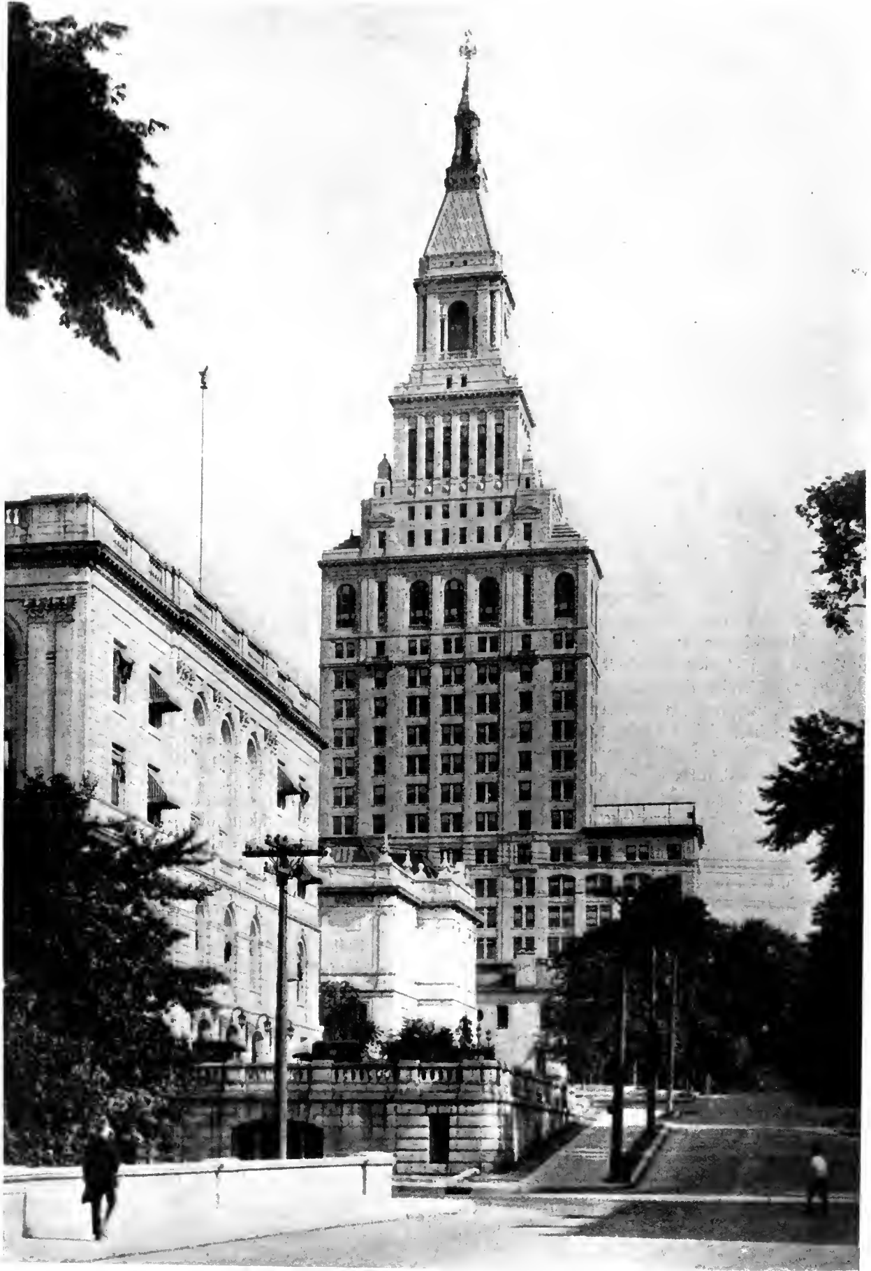
BUILDING OF THE TRAVELERS INSURANCE CO., HARTFORD, CONN. DONN BARBER, ARCHITECT
